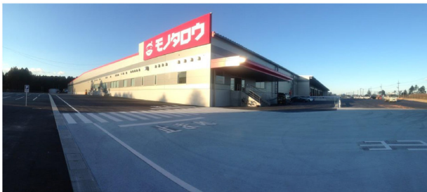
Kasama DC exterior view (Jan. 2017)
