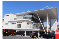
Hybrid Prestressed and Concrete Roofs (Okinawa Prefecture, Japan)
