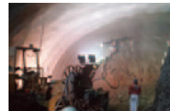
Spraying of tunnel inner walls
