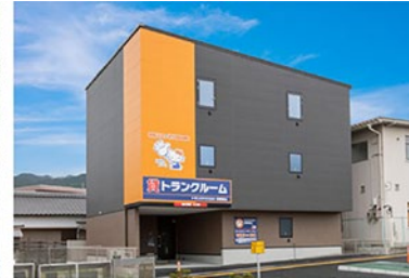
Indoor-type trunk rooms (entire building)
