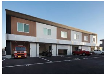
Business storage two-story maisonette
