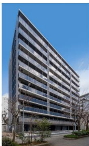
Exterior of building's southwest side
