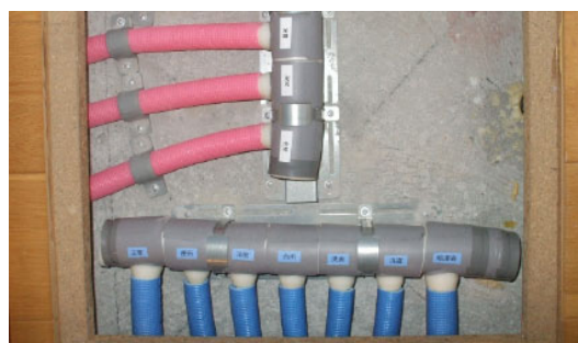
Header pipes
