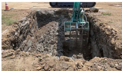
TENOCUBE Method (under construction)
