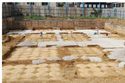
TENOCOLUMN Method (under construction)
