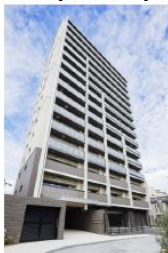
WAKOHRE Fukushima Noda The Residence Fukushima-ku, Osaka (Handover March 2023) No. of units: 56 5 minutes' walk from JR Noda Station
