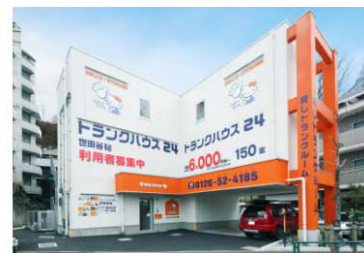
Indoor-type trunk rooms (entire building)
