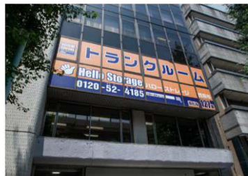
Indoor-type trunk rooms (inside a building)
