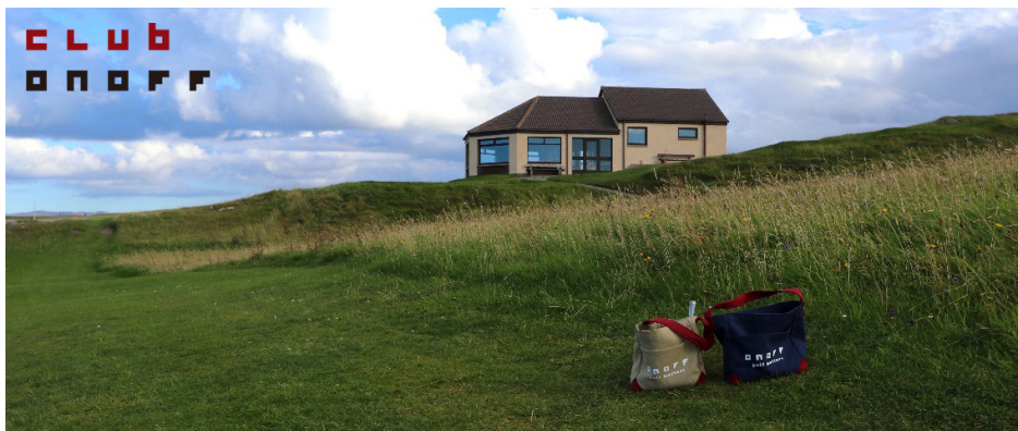
Source: Materials supplied by the Company
