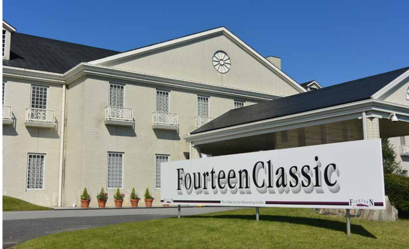
Source: Materials supplied by the Company
