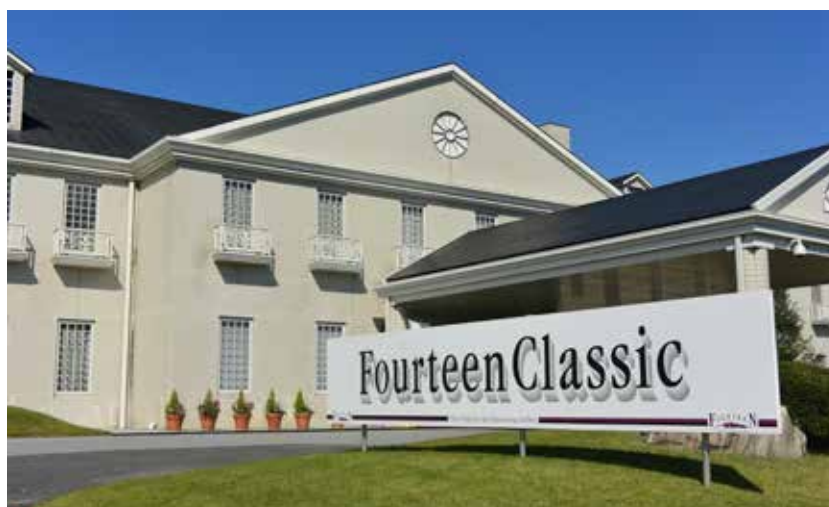
Source: Materials supplied by the Company
